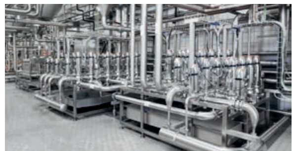
New pressure tank cellar: from manual to automated control – in the cellar, the panel technology was replaced by double-seat valve manifolds.
